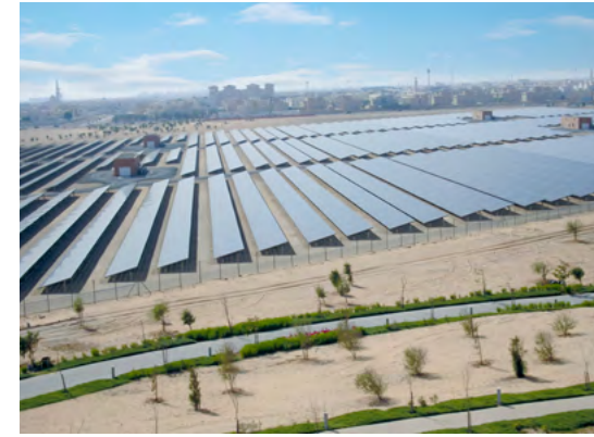
10 MW Solar Farm
