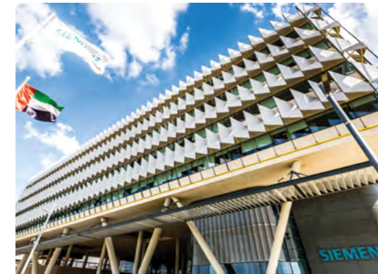
Siemens Middle East HQ at Masdar City
